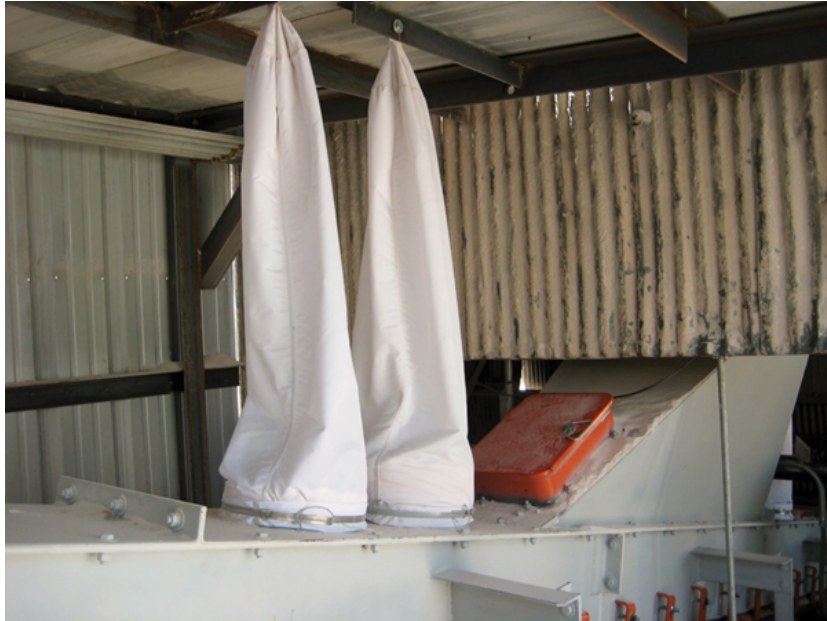
Dust Collector Bags Relieve Excess Air Flow Allowing the Passive System to Control Dust
